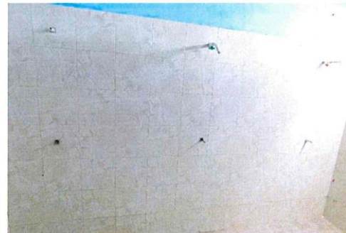
Image 4: Shower with broken fixtures
